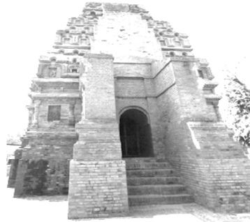
Front View of Bhitargaon Temple Kanpur
